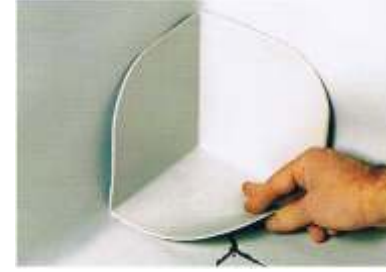
Internal corner treatment
